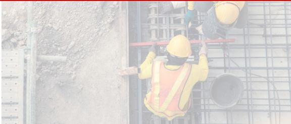
Construction site surveying
